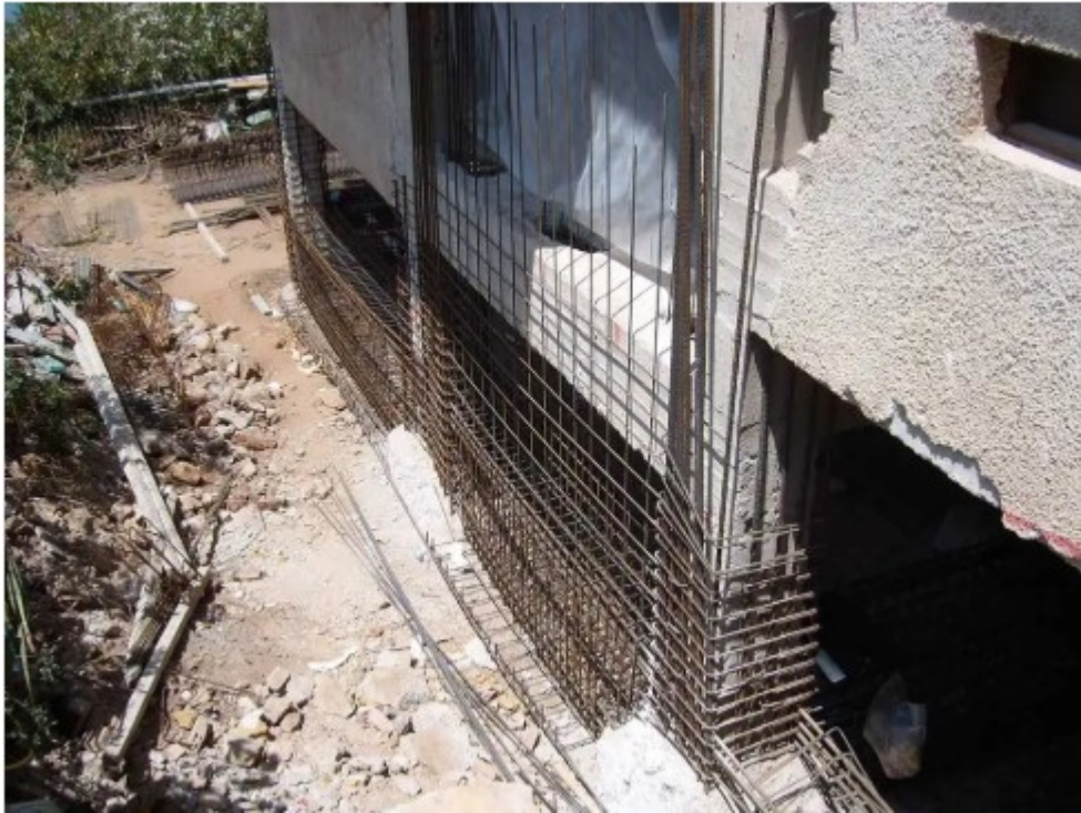
* Adding steel bracing
