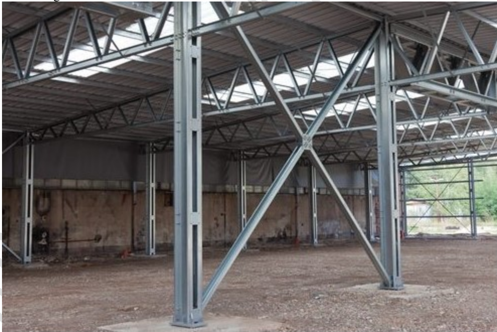
* Strengthening beam-column joints
