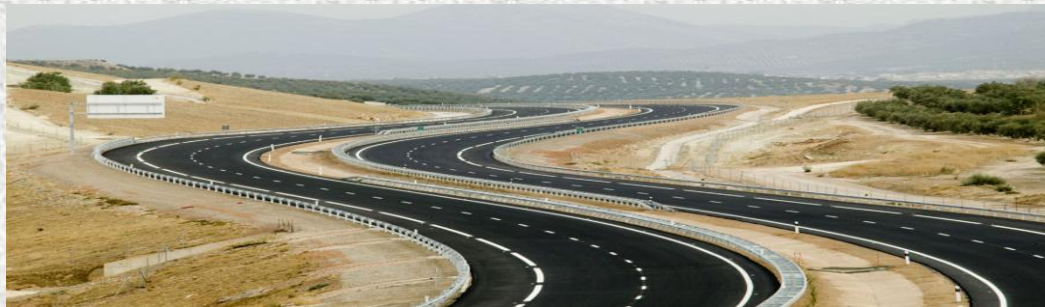
Example: winding alignment in hilly terrain
